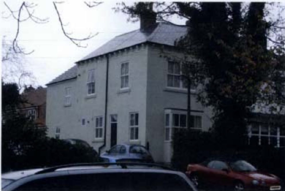
Corner house- Hartburn Village and Frasier road
